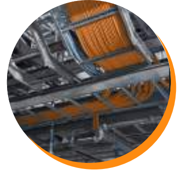
Cable Tray Installation
